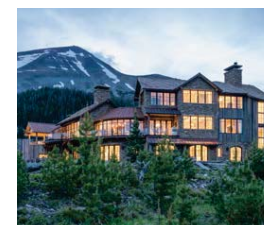
Project: LONE MOUNTAIN HIDEAWAY Architect: JLF Architects
