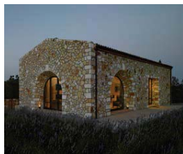
Project: GIESE Architect: Andrew Batey
